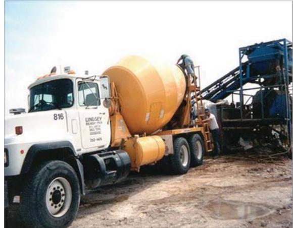
LITEBUILT® FOAM BEING INJECTED INTO CONCRETE TRUCK
