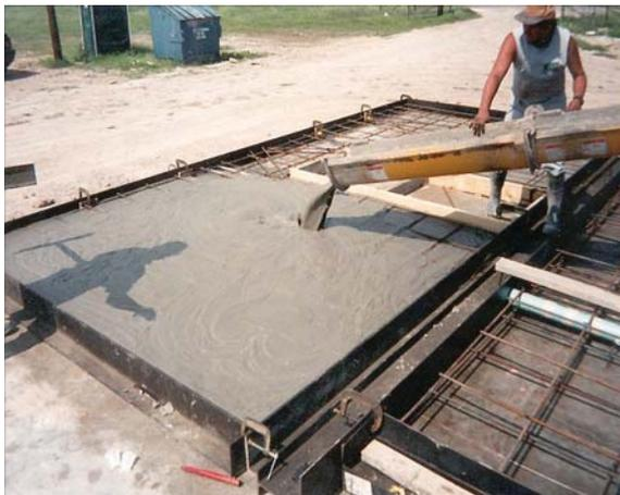
LITEBUILT® AERATED LIGHTWEIGHT PANEL CASTING
